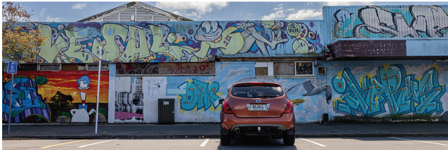
This closed-up building, at 110-114 Seaview Rd in New Brighton is on the city council's list of problem sites. PETER MEECHAM/THE PRESS
