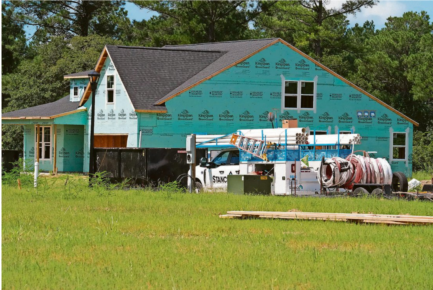
Construction continues in the Trestle Ridge neighborhood of Brunswick Forest on Aug. 31 off of Brisco Way in Leland. KEN BLEVINS/STARNEWS
