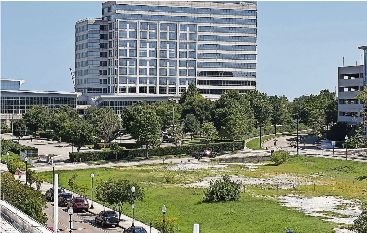
The Skyline Center, shown on July 30, is part of Wilmington's Northern Riverfront Development District. BOB LIEPA/STARNEWS
