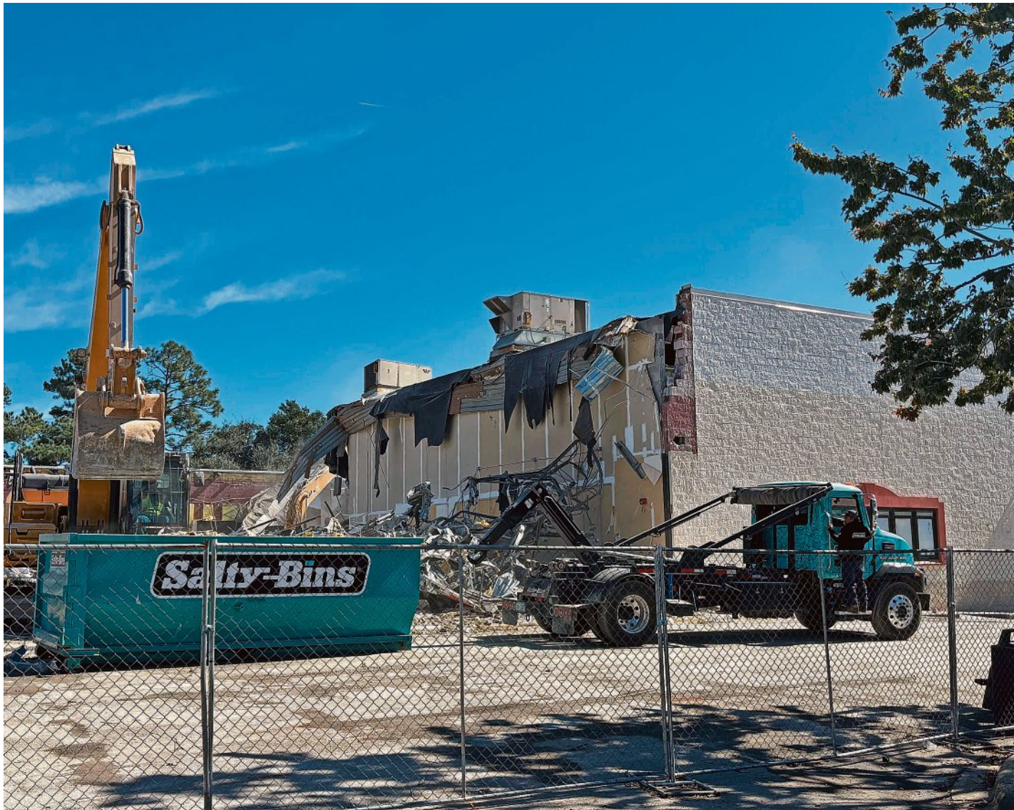
Demolition work on the former AMC Classic 16 cinema at 111 Cinema Dr. in Wilmington continued on Oct. 24 with an excavator dropping debris into a dumpster. PHOTO BY BOB LIEPA/STARNEWS
