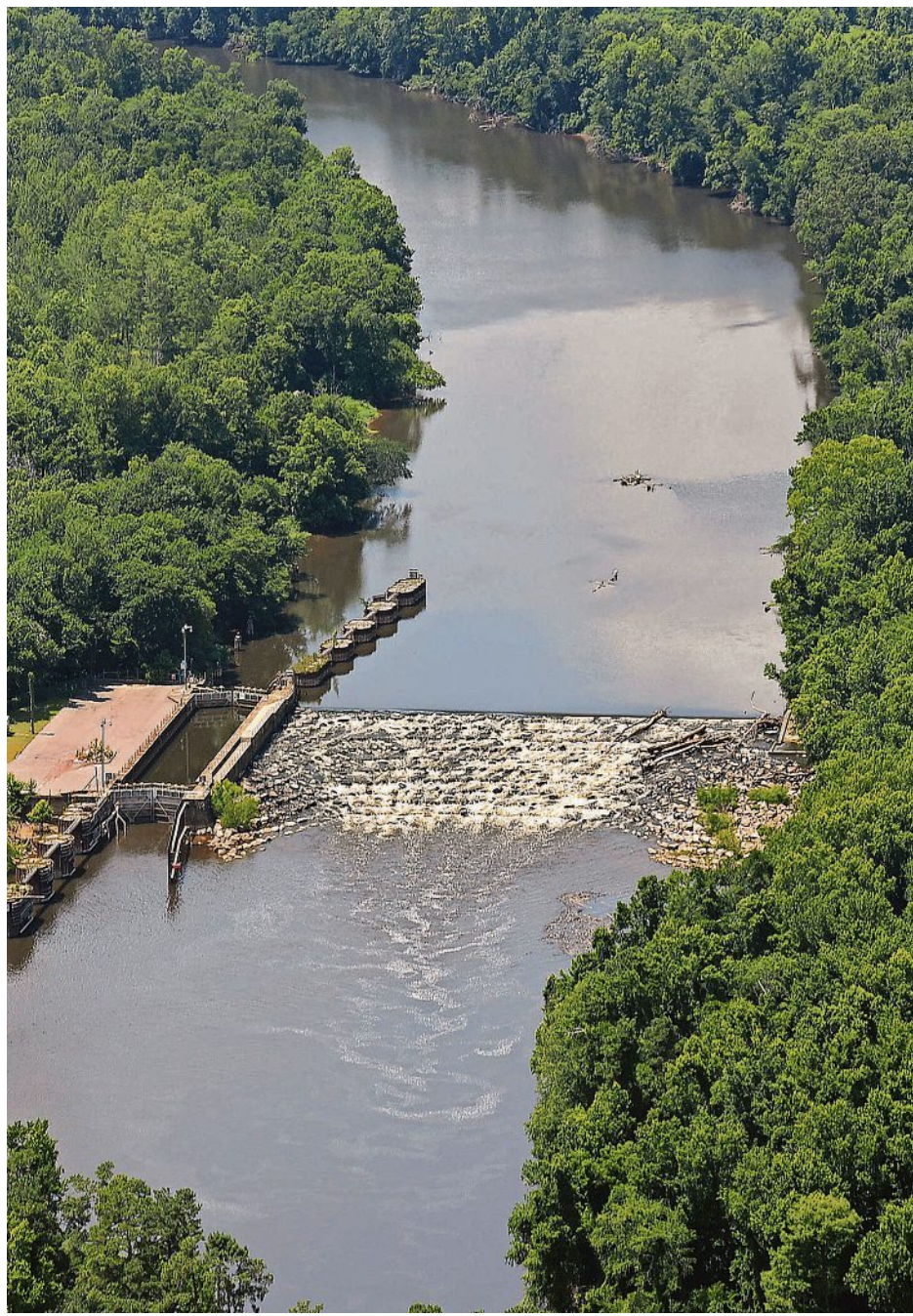
Aerial view of Lock and Dam No. 1 and the rock arch rapids built to help migratory fish get around the structure. KEN BLEVINS/STARNEWS
