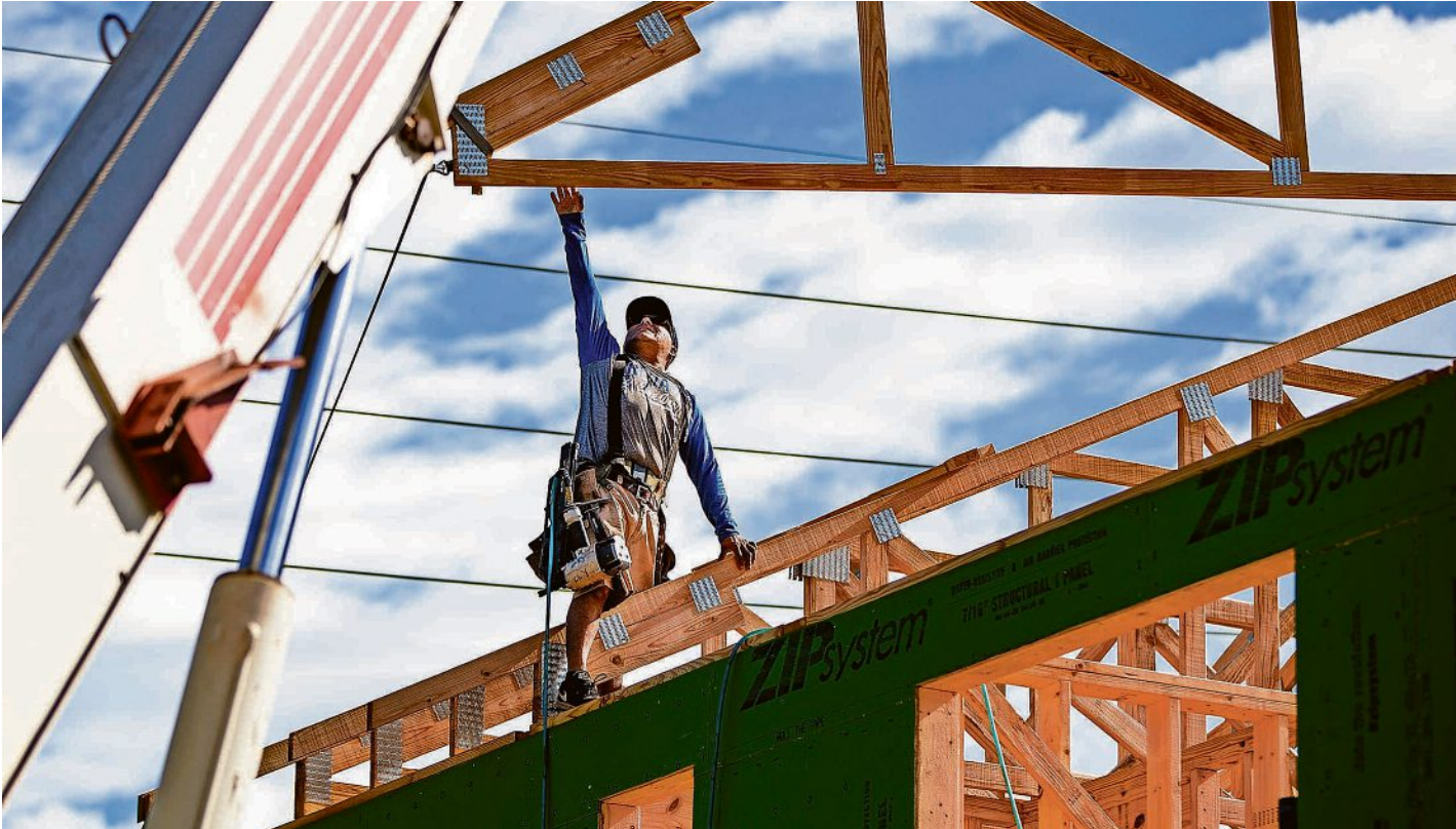
Construction worker Ramiro Martinez guides a roof truss into place atop a new house under clear skies along Edwards Avenue in Asheville on July 2.
