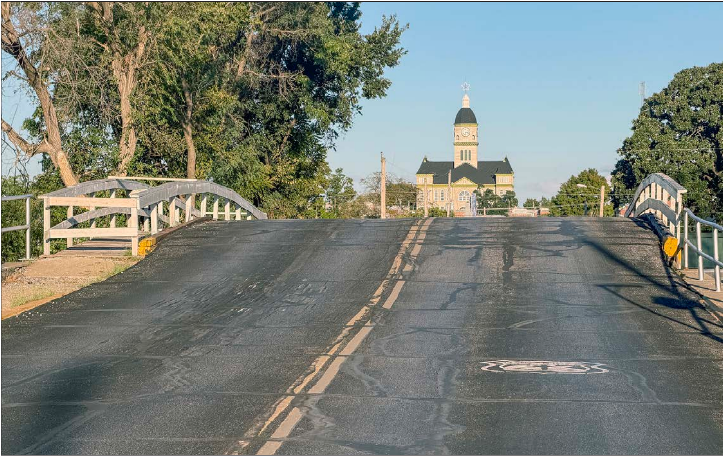
This view shows the change in slope at the top of the Oak Street bridge in Carthage.
