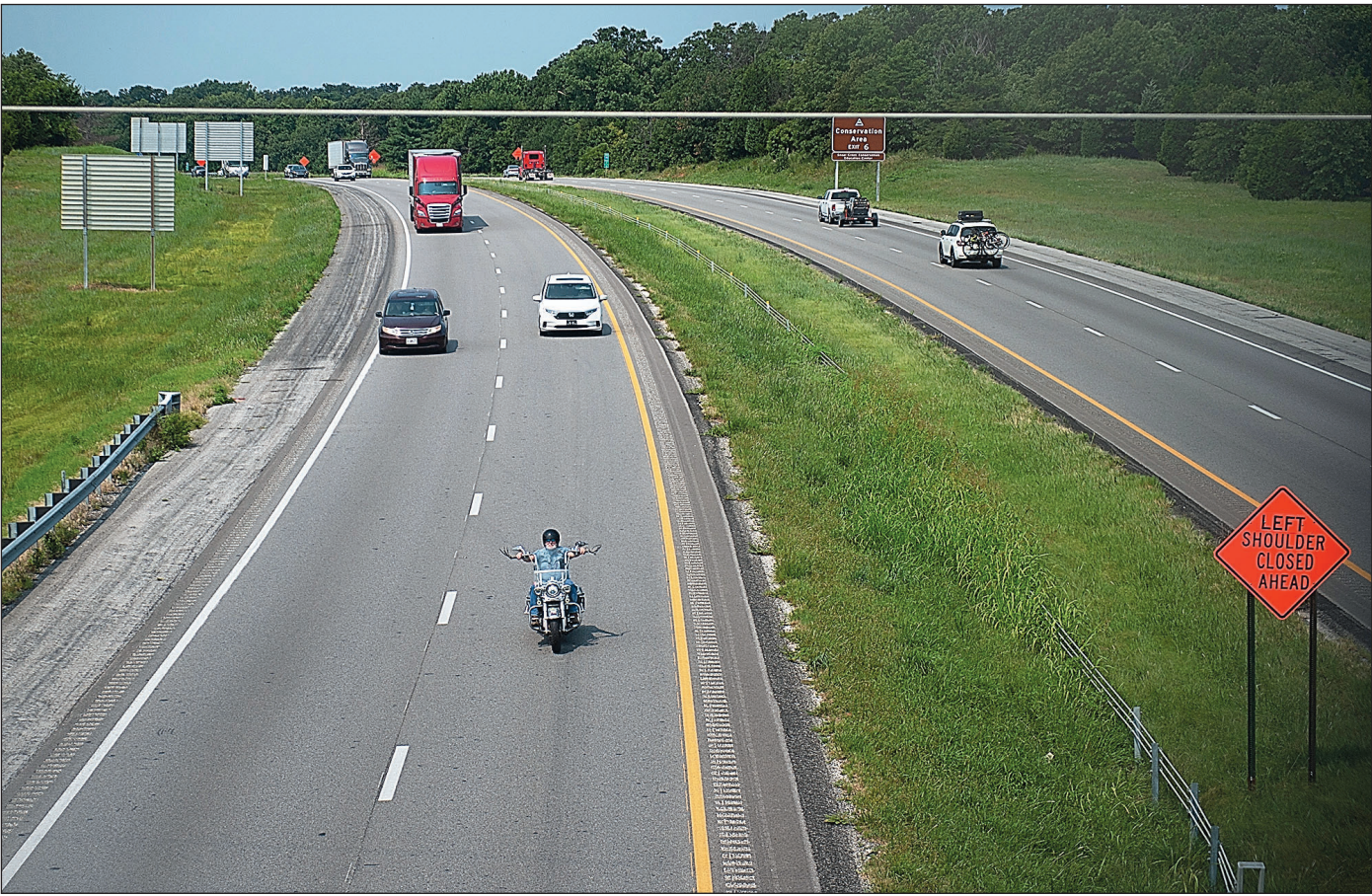
Traffic travels under the Connecticut Avenue bridge on Interstate 44. A groundbreaking will be held later this month for Forward 44, bringing improvements valued at a half-billion dollars.
