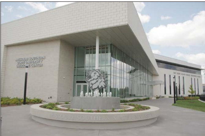
The "new front door" to Missouri Southern State University is the two-story side of the newest building on campus. Enrolling MSSU students will visit places such as admissions and the registrar's office inside the Roy Blunt Health Science Innovation Center. GLOBE FILE
