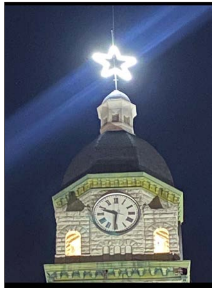
The Peace Star on top of the Jasper County Courthouse in Carthage shines brightly after it was removed for repairs then put back up when those repairs were finished.
