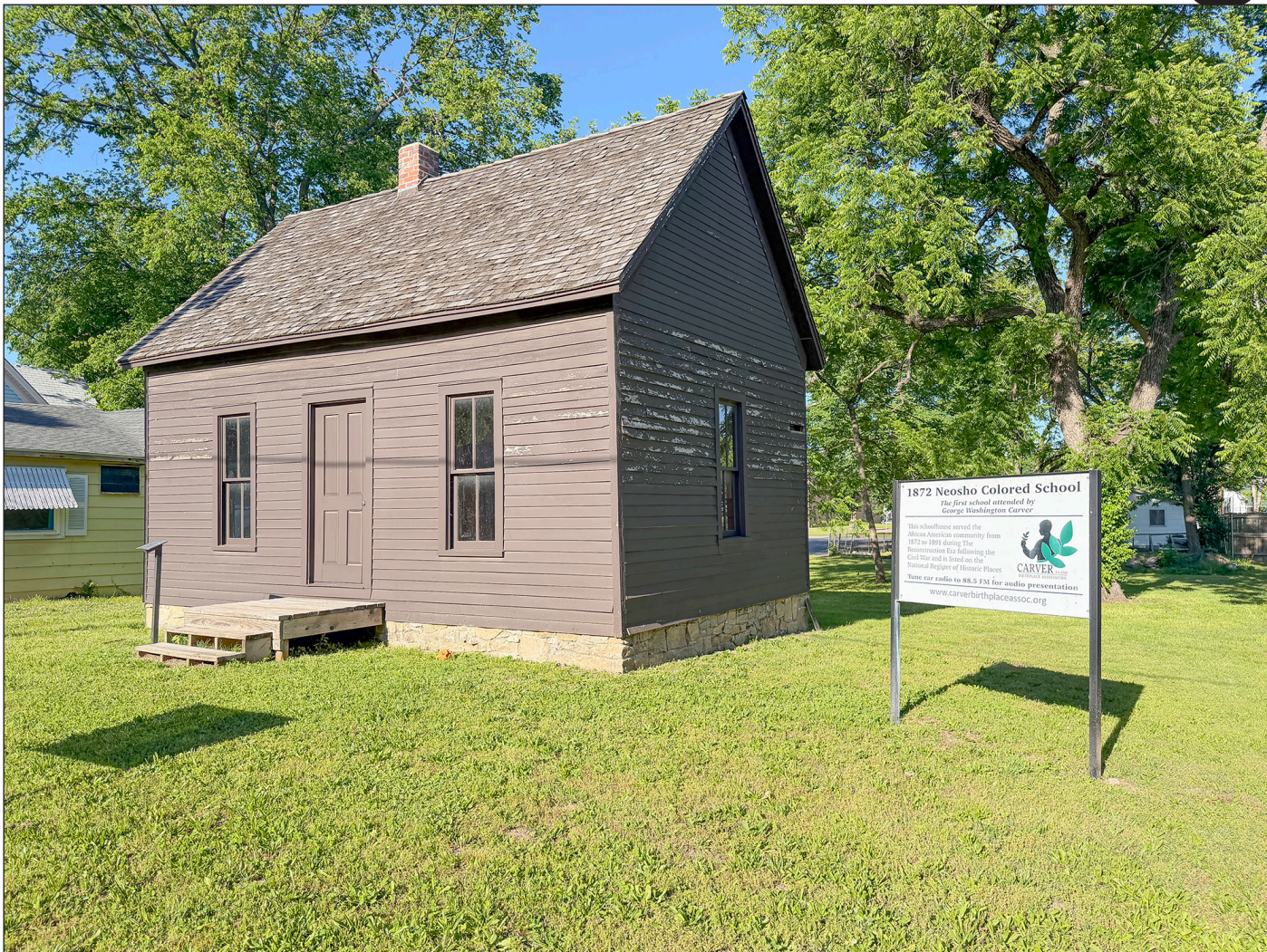
Work will begin in the next few days on interior renovations of the former Neosho Colored School at 639 Young St. in Neosho.
