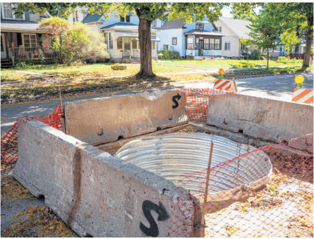
DILAN PAREKH • For the Minnesota Star Tribune A hole at the intersection of 30th and 33rd avenues in Minneapolis. The city is upgrading 17 miles of aging water main cast iron pipes.
