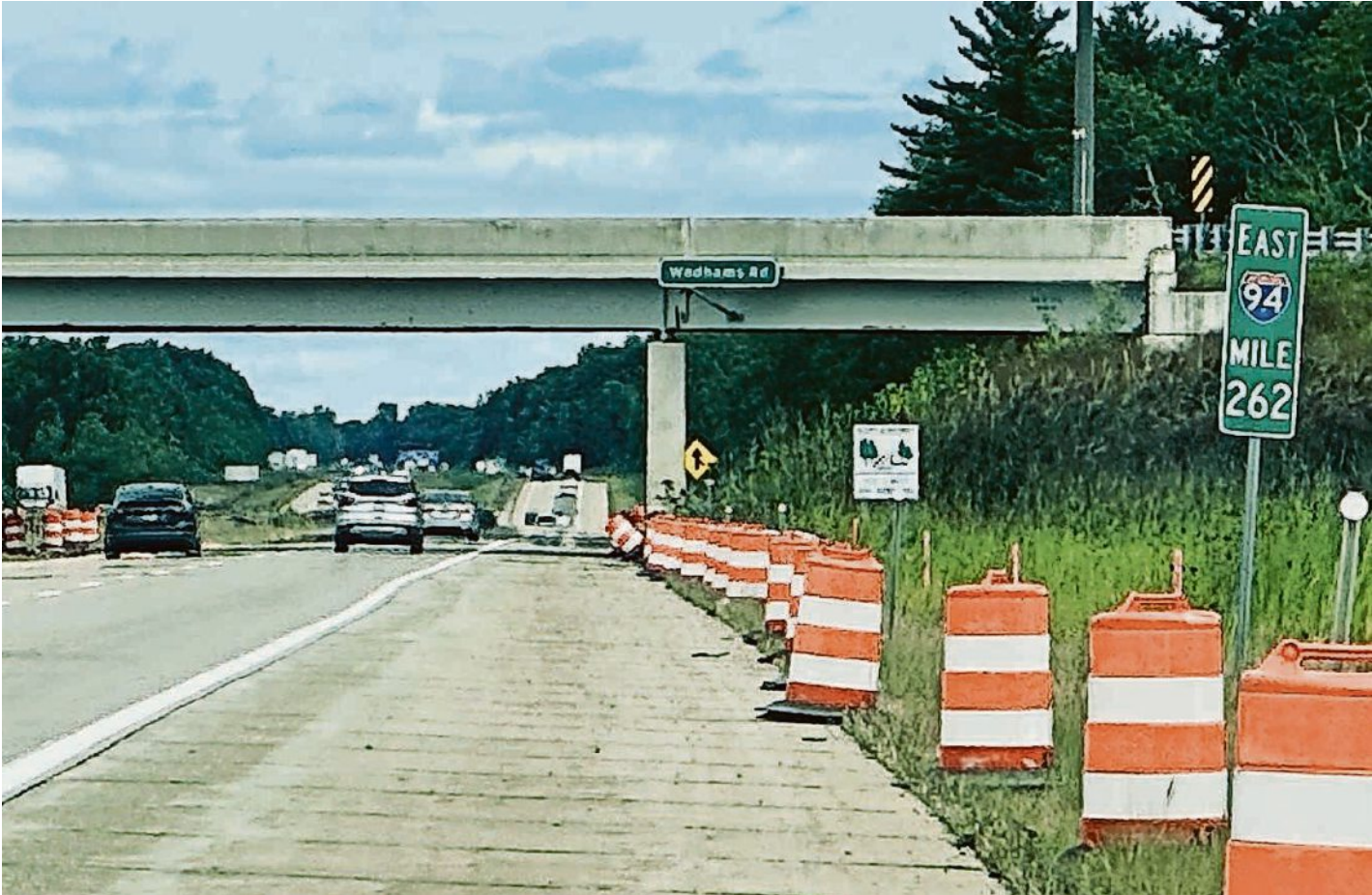
A weeklong road work schedule outlines full closures and lane restrictions across multiple St. Clair County townships.
