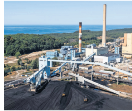
In just over four months, Consumers Energy ran up $80 million in net costs to keep its coal-powered J.H. Campbell Generating Complex in Ottawa County on life support, the utility disclosed in a Thursday regulatory filing. MLive.com files
