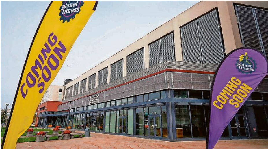
The site at of a new Planet Fitness at The Heights building on Oct. 13.
