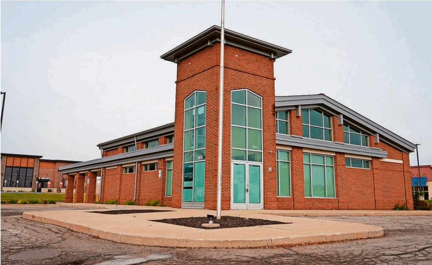
The future site of Chick-Fil-A on Oct. 13 near the Eastwood Towne Center in Lansing Township. The former Comerica Bank building will be demolished to make way for the restaurant. PHOTOS BY NICK KING/LANSING STATE JOURNAL
