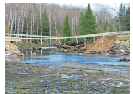
A drained Bucks Pond is all that's left after the dam near Barton City failed on April 13 after heavy rains and snowmelt. Sheri McWhirter, MLive.com
