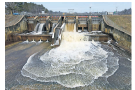
Rogers Dam on the Muskegon River is one of 13 dams that Consumers Energy wants to sell to Confluence Hydro, a subsidiary of a private equity firm.
