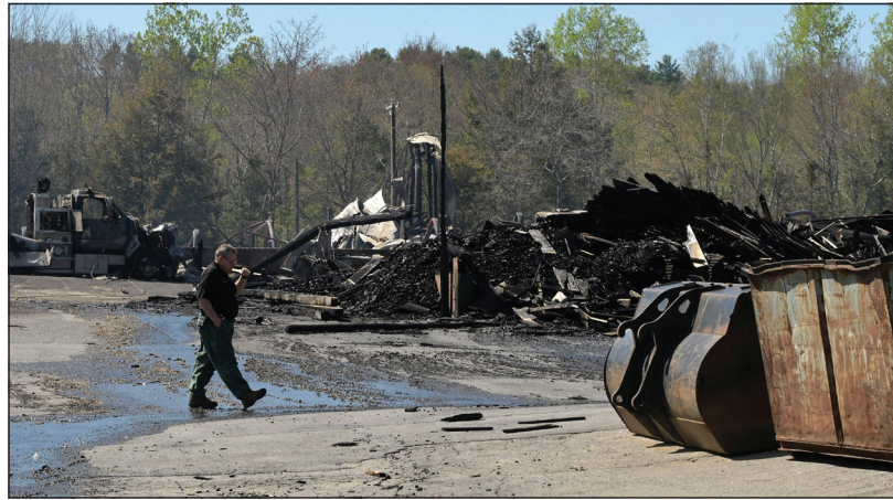
A man walks past a burned out fire truck, left, and an incinerated structure at Robbins Lumber in Searsmont on Saturday. Federal agents have joined the investigation into the fire and explosion's cause. (RICH ABRAHAMSON/STAFF PHOTOGRAPHER)
