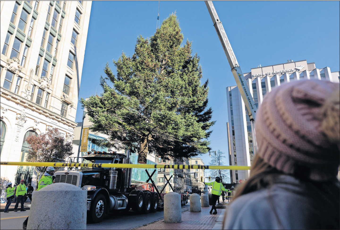
Freya Rice, 4, watches as her dad, Cody Rice, operates the crane lifting the holiday tree into place in Portland’s Monument Square on Wednesday. Freya and her siblings came down from Lewiston with Rice’s fiancée to watch the delicate operation. The city’s tree-lighting ceremony is planned for the evening of Nov. 28. (BRIANNA SOUKUP/STAFF PHOTOGRAPHER)
