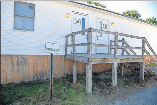
At George E. Jack School in Standish, portable classrooms are still in use years longer than intended. (DARYN SLOVER/STAFF PHOTOGRAPHER)
