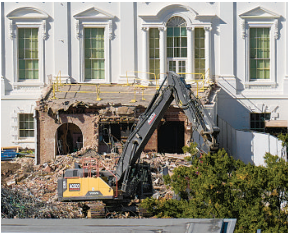
Demolition continued Thursday on a portion of the East Wing of the White House in preparation for the construction of a new ballroom. Montgomery County company Aceco's logo is visible on the equipment, leading to backlash from those who oppose the project.
