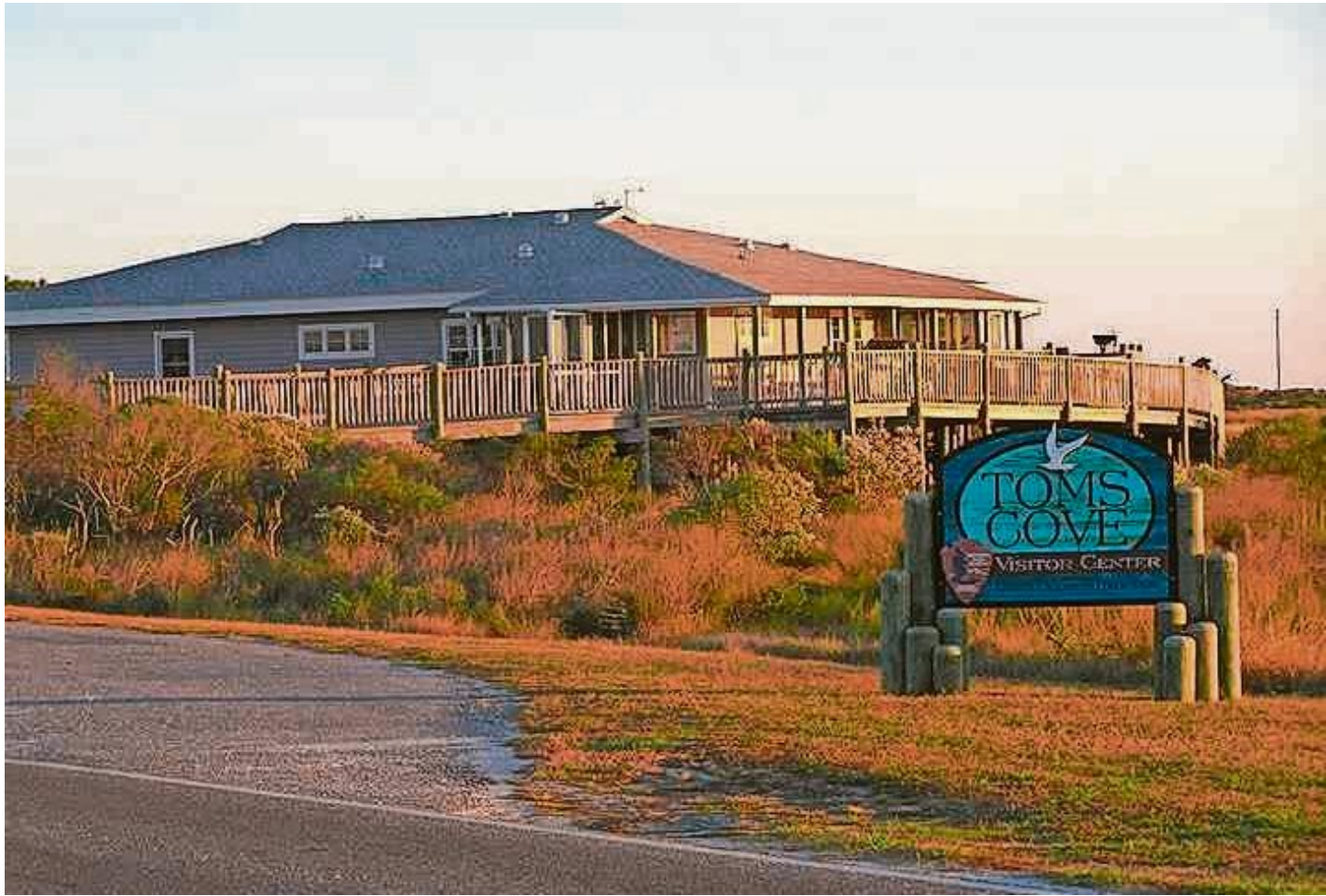
The Tom’s Cove Visitor Center building in the Virginia Unit of Assateague Island National Seashore has now closed permanently and is set for demolition in early January 2026. PHOTO PROVIDED BY ASSATEAGUE ISLAND NATIONAL SEASHORE
