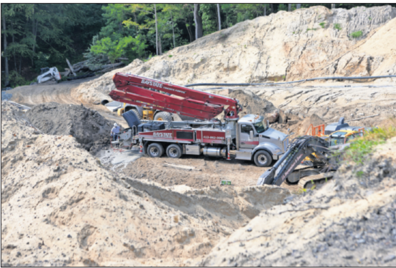
Springfield officials tour a $2.5 million culvert repair project at the entrance road to Forest Park connecting with Swan Pond in 2019. (DON TREEGER / THE REPUBLICAN FILE)
