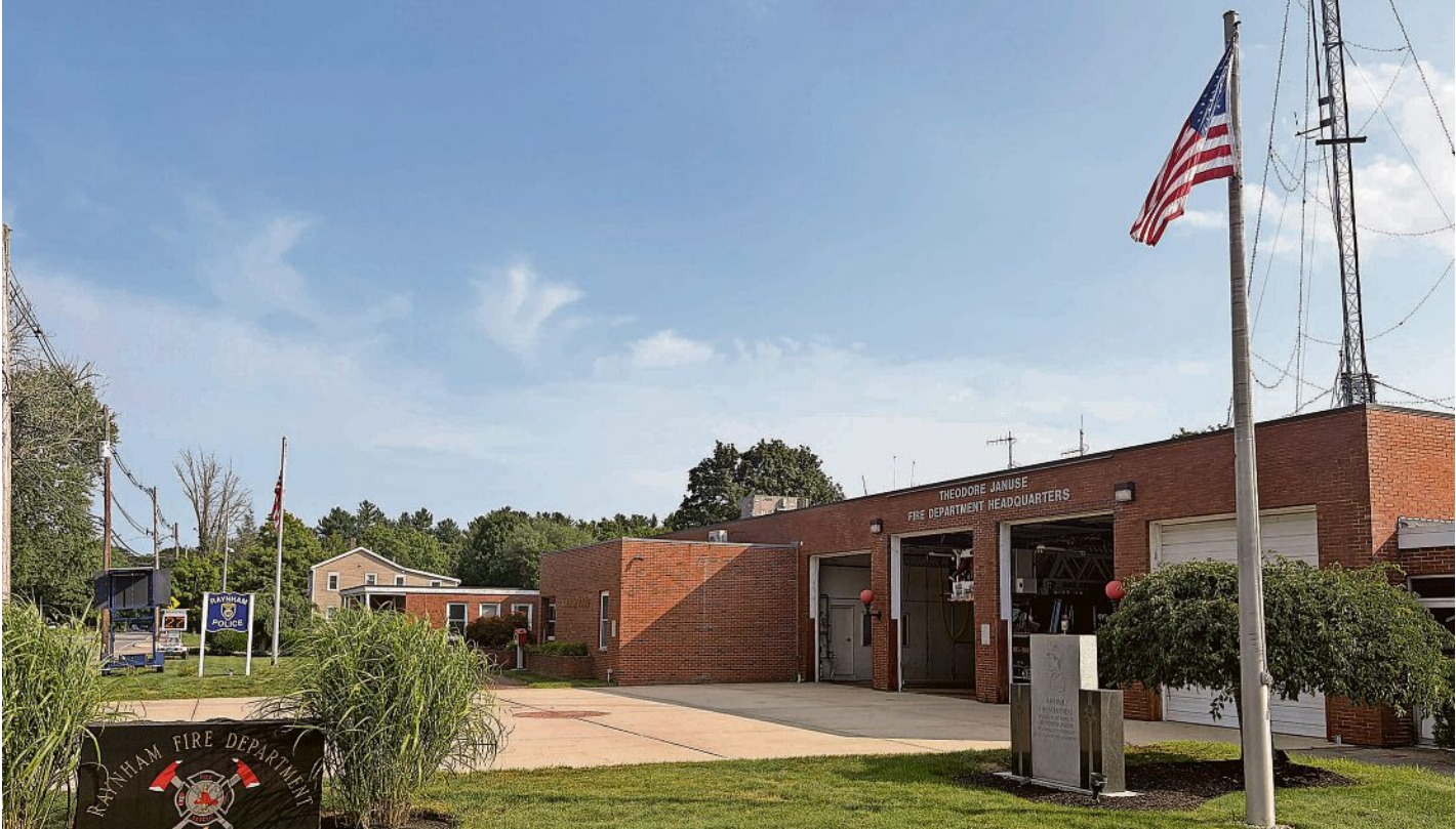
The town plans to replace Raynham’s current fire and police stations on Orchard Street, seen here on Aug. 10, with a new public safety building on the same site. DANIEL SCHEMER/TAUNTON DAILY GAZETTE
