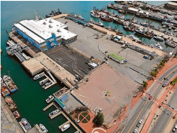
The state is going to close State Pier’s south wharf and most of the east wharf within weeks for significant repairs that will cause the displacement of virtually all water-dependent businesses.
