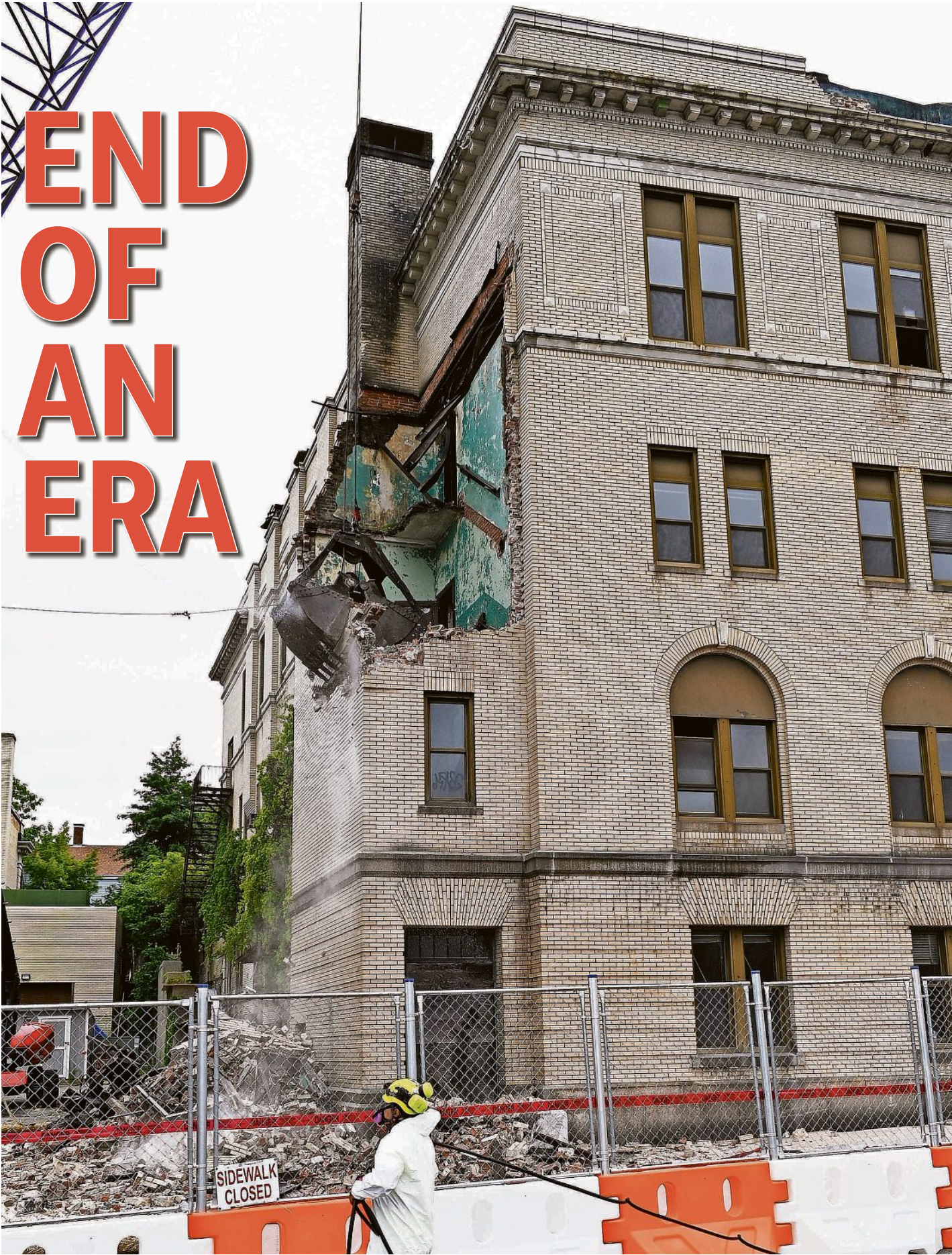
The demolition of the old Fall River police station on Bedford St. began on August 18. PHOTOS BY COLIN FURZE/HERALD NEWS
