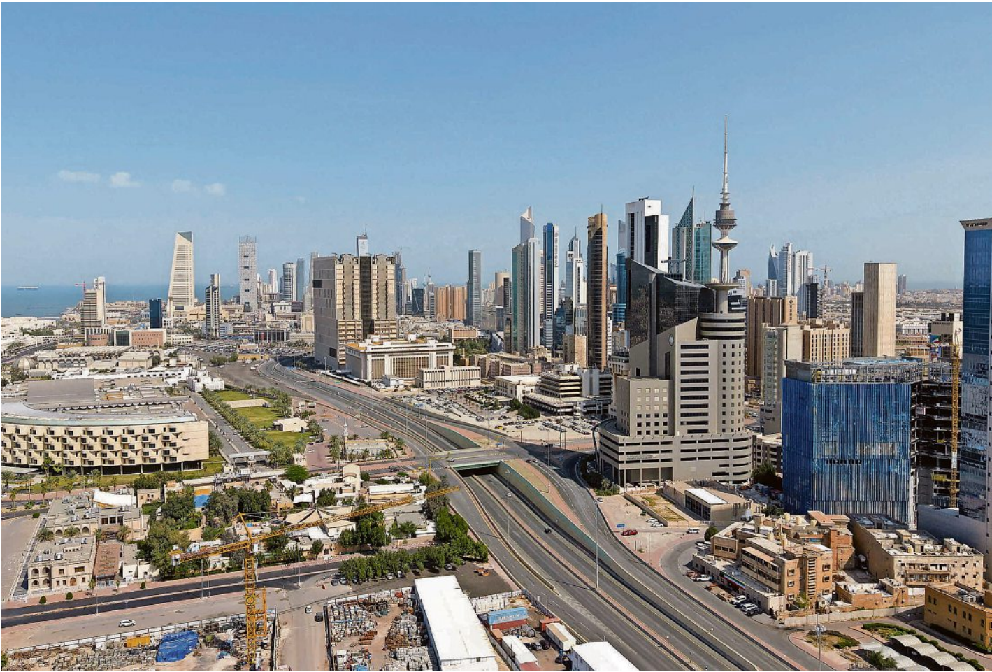
Authorities in Kuwait said one of its power generation and water desalination stations had been hit in an Iranian attack. STEPHANIE MCGEHEE/REUTERS FILE
