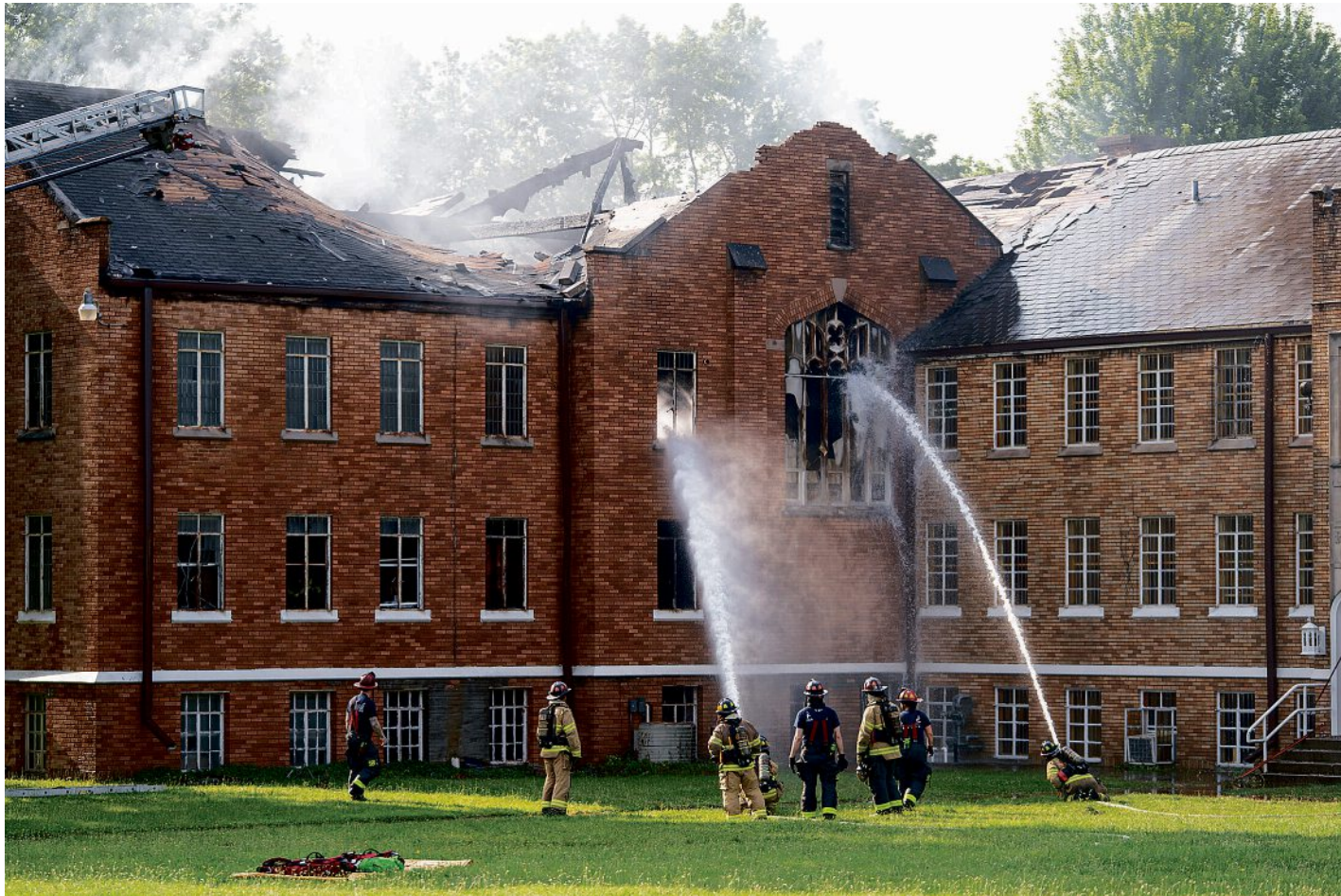
The South Bend Fire Department battles a fire July 6 at Maranatha Fellowship 7th Day Sabbath Church on Ewing Avenue in South Bend. MICHAEL CLUBB/SOUTH BEND TRIBUNE
