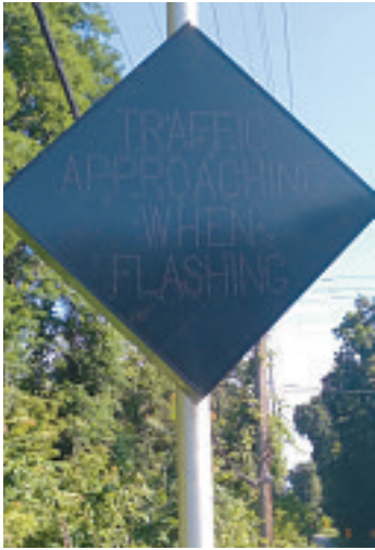
A new warning sign is being installed at the intersection of Waverly Road and U.S. 12. JIM WOODS/FOR THE POST-TRIBUNE
