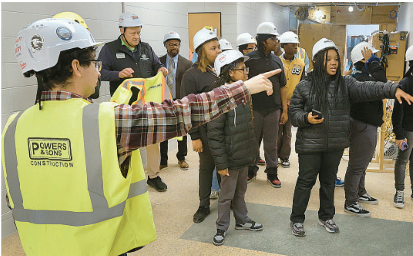
Saul Alvarez, project engineer for Powers and Sons Construction, left, and student Sharaya, 12, point out locations at the job site of the Tolleston Opportunity Campus in Gary Wednesday, April 8, 2026. JOHN SMIERCIAK/FOR THE POST-TRIBUNE
