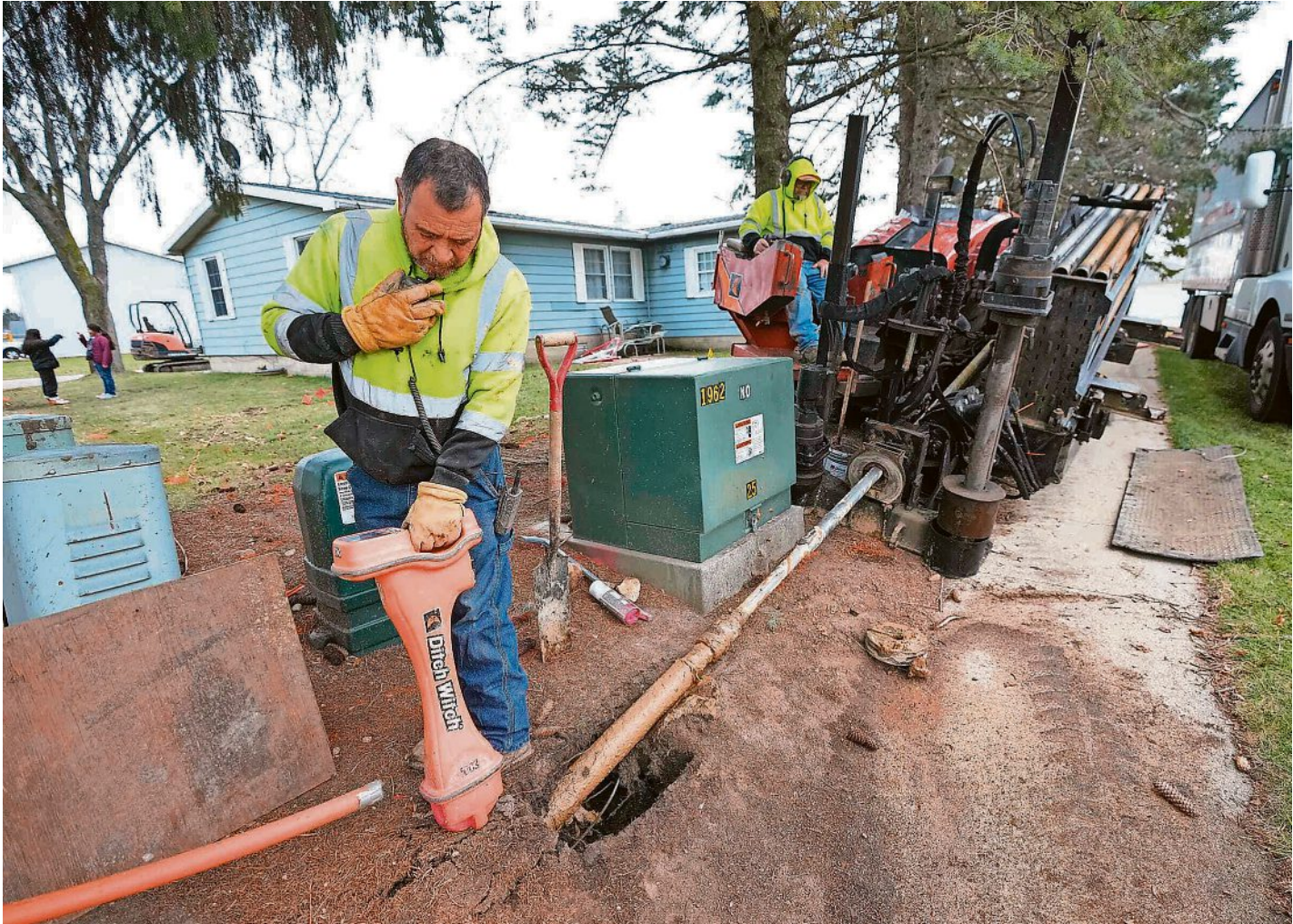
Sal Martinez (left), a directional bore drill locator and Chris Halvorson, a foreman with Northwest Cable Construction, Inc. out of Mayville, contracted by TDS Telecom, work on drilling holes for duct work that will eventually house broadband internet cable in the Easttown Manor subdivision of Elkhorn on Dec. 5, 2022. MIKE DE SISTI/MILWAUKEE JOURNAL SENTINEL
