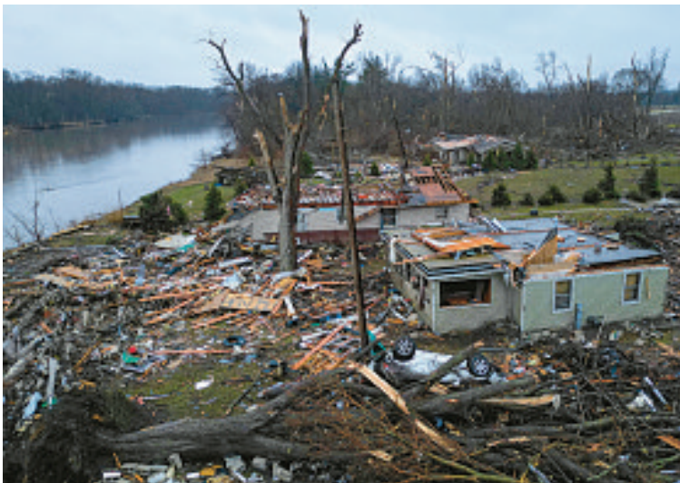
Debris lies on the ground on March 11 after a tornado struck the evening before along South Sandbar Road in Aroma Park. The homes border the Kankakee River. STACEY WESCOTT/CHICAGO TRIBUNE
