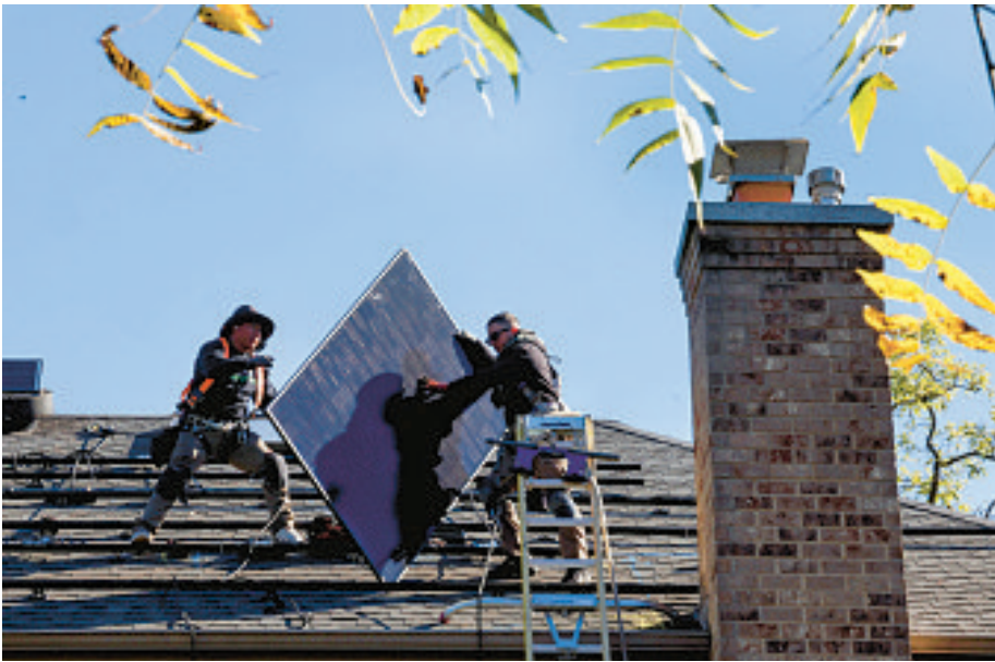
Workers Danny Satay, left, and Ivan Casiano install solar panels on a home in Elmhurst on Friday. STACEY WESCOTT/CHICAGO TRIBUNE
