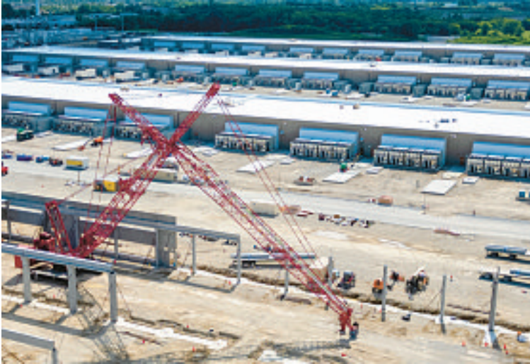
Construction at the new Compass Datacenters 197-acre site in Hoffman Estates on June 23. Compass is constructing five hyperscale data centers on the former Sears Headquarters campus. STACEY WESCOTT/CHICAGO TRIBUNE
