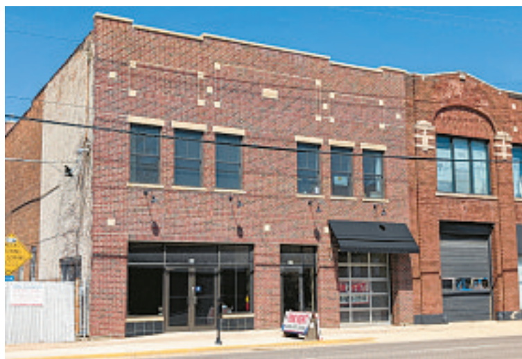
The building at 55 S. Lake St. in Aurora, the former location of Warehouse 55, soon will hold Superjumbo Records and Arcade. R. CHRISTIAN SMITH/THE BEACON-NEWS
