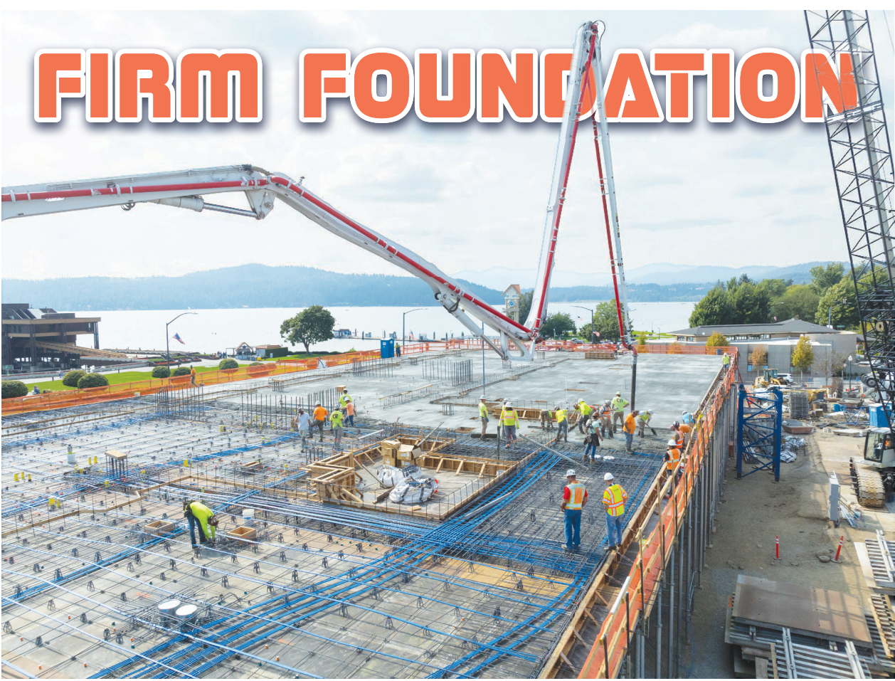
Interstate Concrete poured 800 cubic yards of concrete for the second floor of Sherman Tower on Friday — the largest pour of the entire project.
