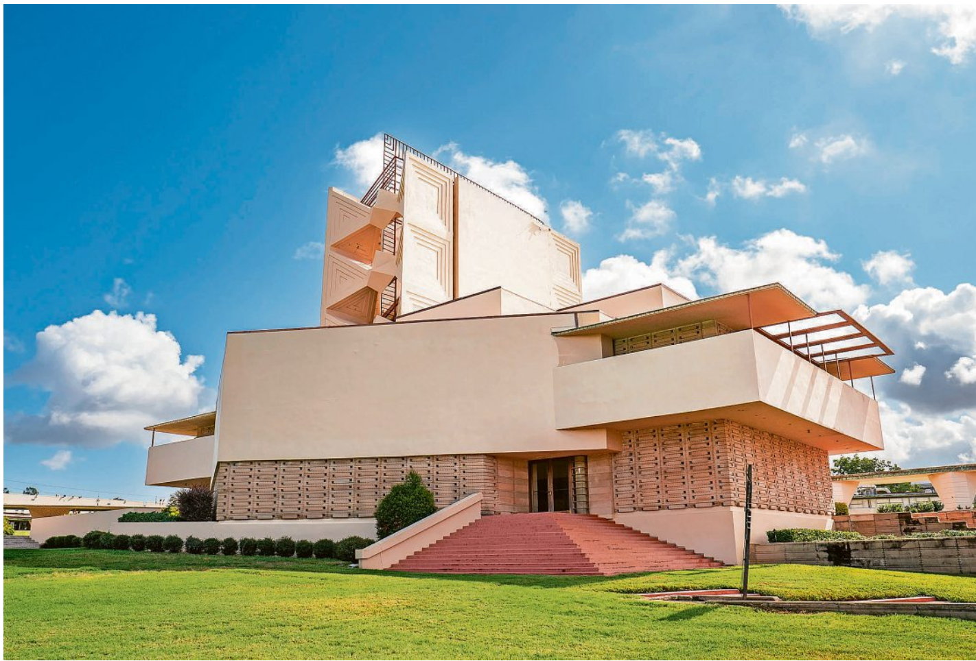
Crews have completed repairs to the roof of Annie Pfeiffer Chapel at Florida Southern College, returning the exterior to its "monochromatic" appearance, as FSC President Jeremy Martin described it. PROVIDED BY FLORIDA SOUTHERN COLLEGE
