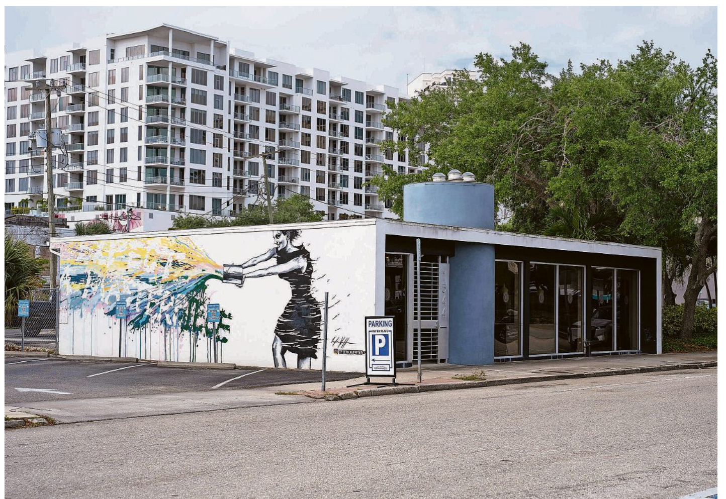
The city of Sarasota bought this building at 1544 First St. for $2.1 million in September 2024, with a plan to use the land as part of an attainable housing complex. PHOTOS BY EARLE KIMEL/SARASOTA HERALD-TRIBUNE
