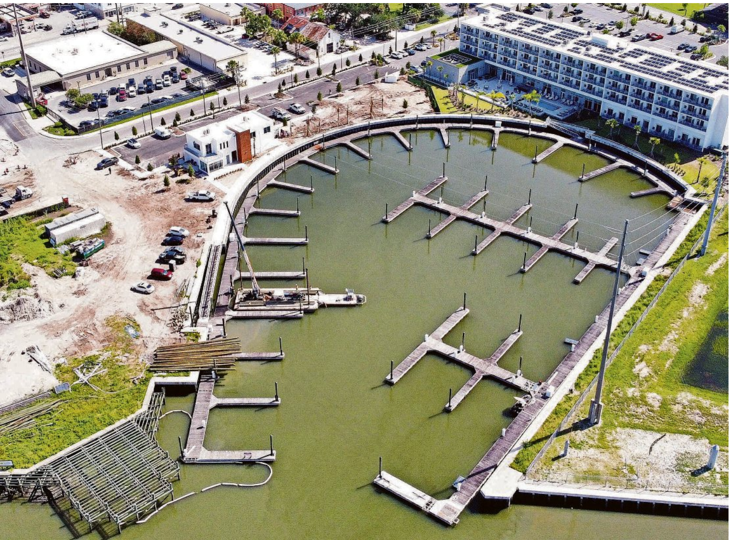
St. Augustine's Sebastian Harbor Marina, a 64-slip boutique marina situated on the San Sebastian River bordering AC Hotel by Marriott St. Augustine, is expected to open in October. PHOTOS PROVIDED BY SEBASTIAN HARBOR MARINA
