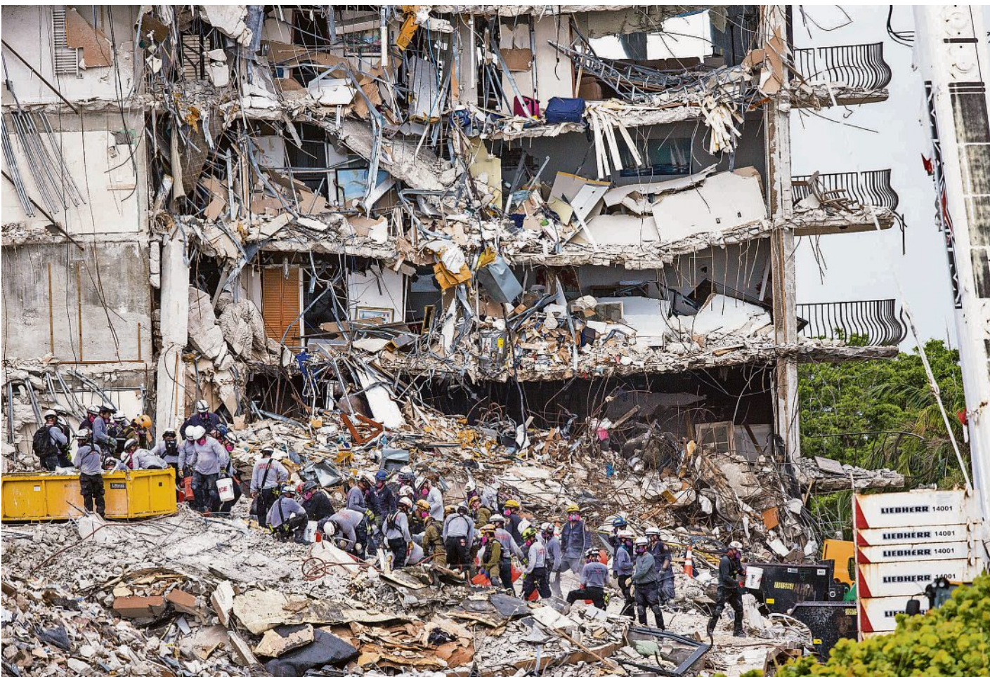
Rescuers search through the rubble of the Champlain Towers South condo collapse in Surfside on June 29, 2021. The National Institute of Standards and Technology announced June 22, 2026, that the structural failure started three weeks earlier at two garage columns. PHOTOS BY ANDREW WEST/FORT MYERS NEWS-PRESS
