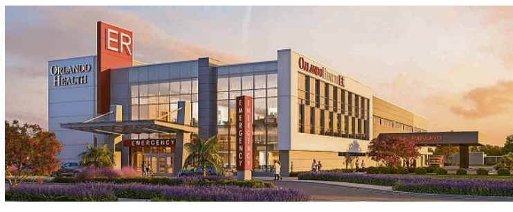
An artist's rendering shows a planned Orlando Health Viera hospital expected to break ground in June. PROVIDED BY ORLANDO HEALTH
