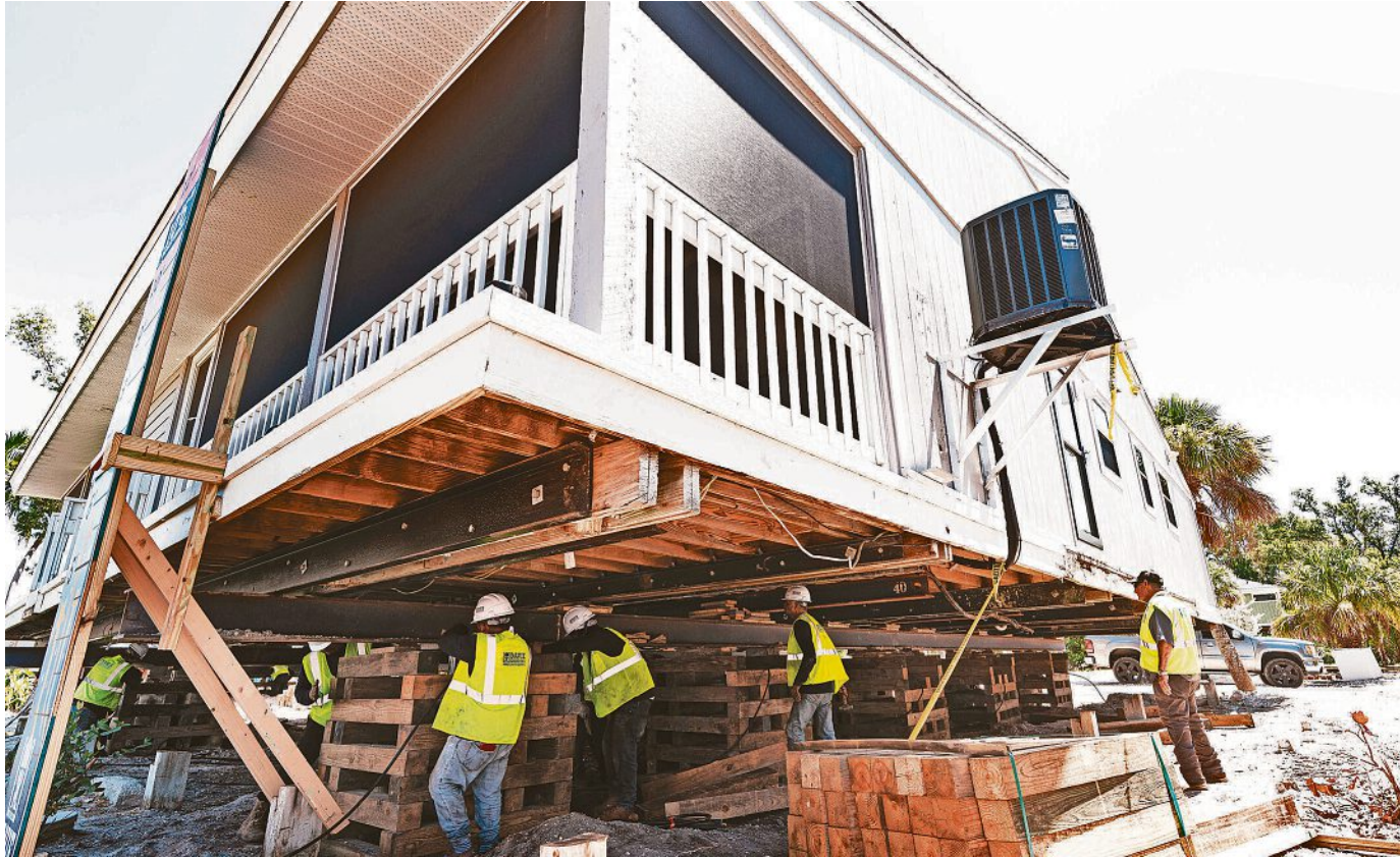
Crews from Davie Shoring work to elevate 11 structures from Donax Village on Sanibel on Aug. 4. The homes were impacted by recent hurricanes that include, Ian, Helene and Milton. The structures will be raised 11 feet over the course of the project, with most of the lifting happening on Aug. 4. ANDREW WEST/THE NEWS-PRESS
