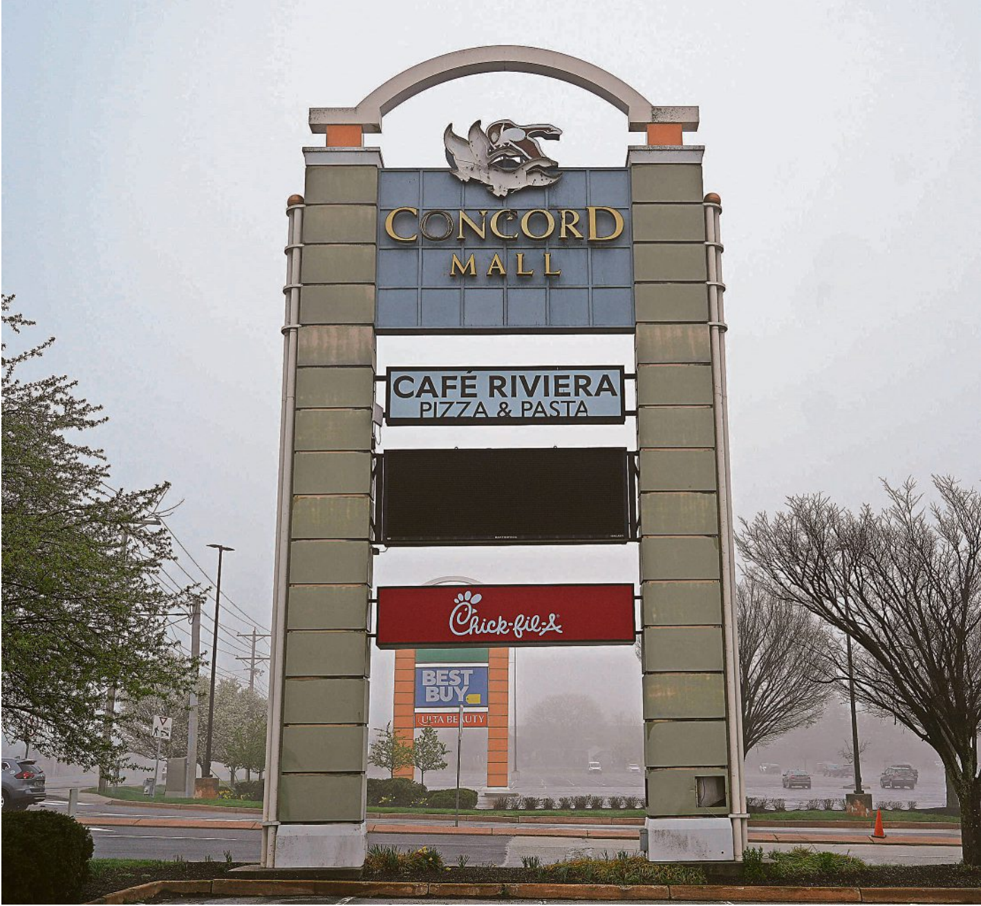
An application has been filed to demolish Concord Mall in Brandywine Hundred. DAMIAN GILETTO/DELAWARE NEWS JOURNAL
