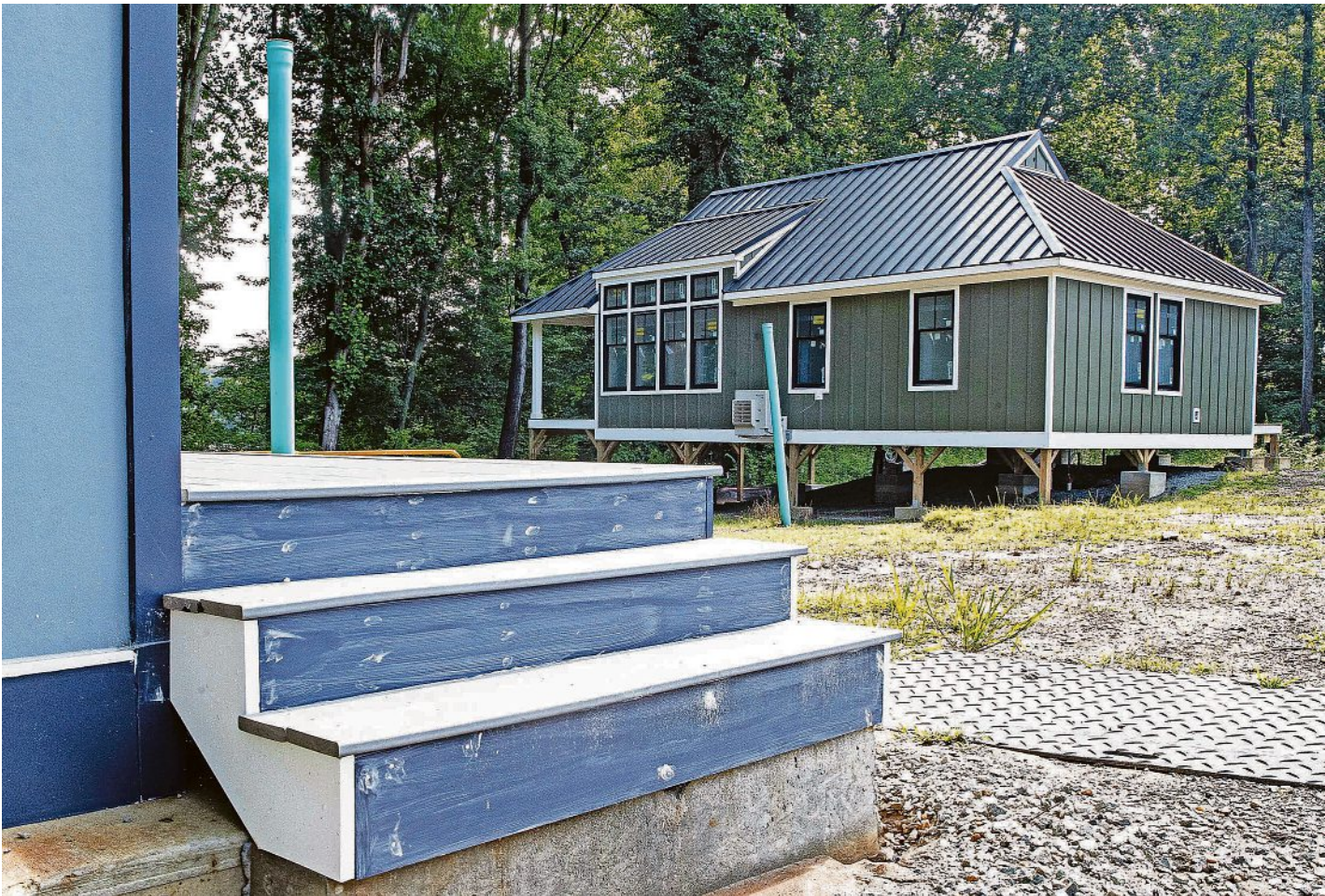
Cabins under construction are seen at Lums Pond State Park near Glasgow on July 29.
