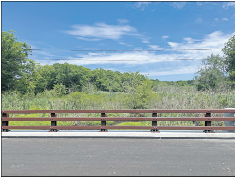
KIMBERLY DRELICH/THE DAY The new Quaker Farm Road Bridge over Haley’s Brook is seen Friday. Structural problems closed the previous bridge in 2018.
