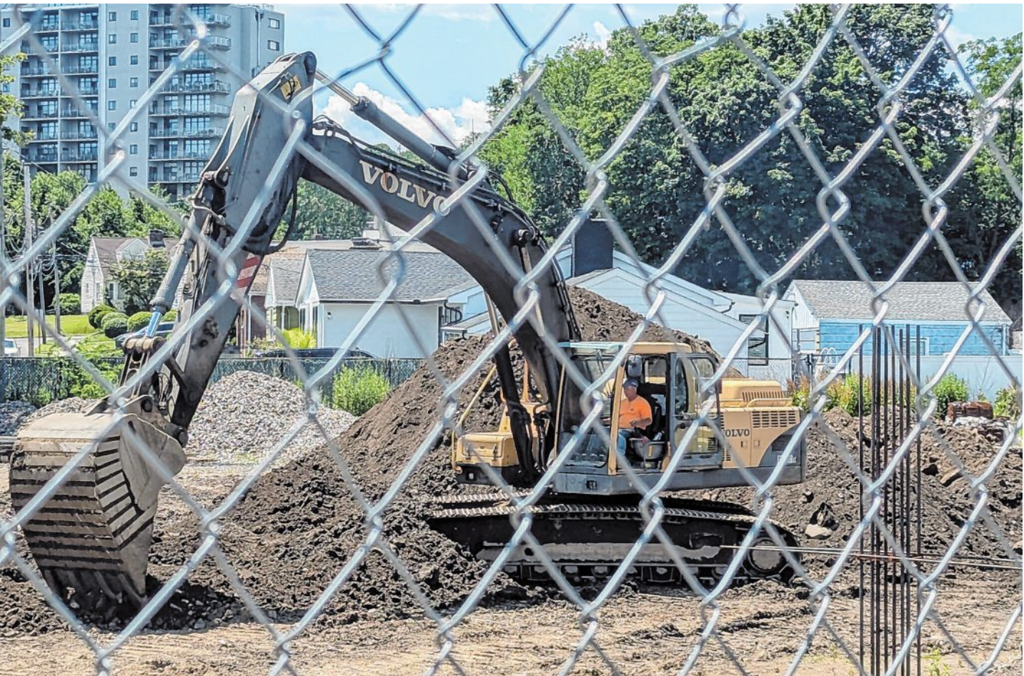
Photos by Brian Lockhart/Hearst Connecticut Media Work resumes Wednesday on an apartment complex at the former Testo's restaurant property in Bridgeport's North end.
