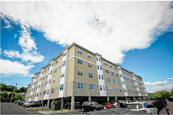
Cedar Village at the Locks, a new apartment development on Canal Street in Shelton.
