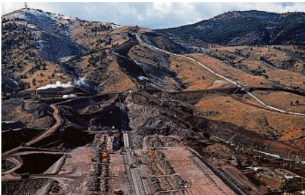
The construction of the main dam of Northern Colorado's newest reservoir, Chimney Hollow Reservoir, is seen from an overlook near Loveland on Feb. 22, 2024. The reservoir is expected to be completed in 2025. LOGAN NEWELL/THE COLORADOAN
