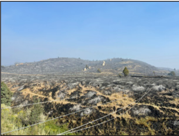
Photos courtesy of WHITE RIVER ELECTRIC ASSOCIATION Power lines lie on the ground after wildfires burned in Rio Blanco County this summer.
