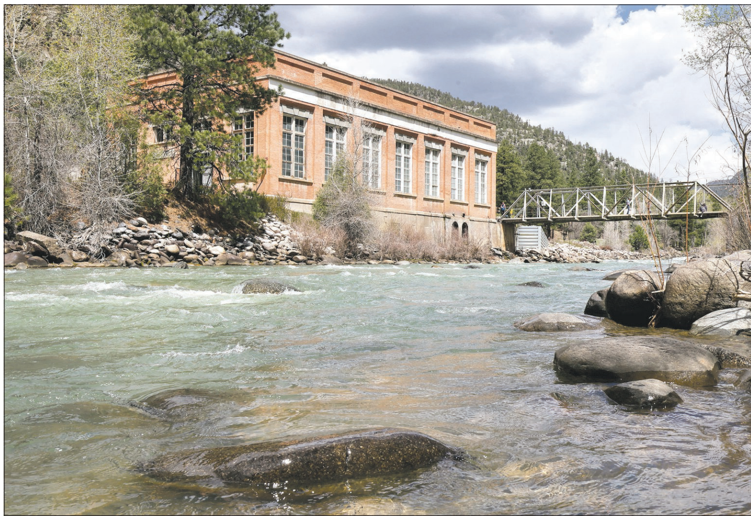
The Tacoma Generation Station along the banks of the Animas River started generating hydro power in 1906 north of Durango.
